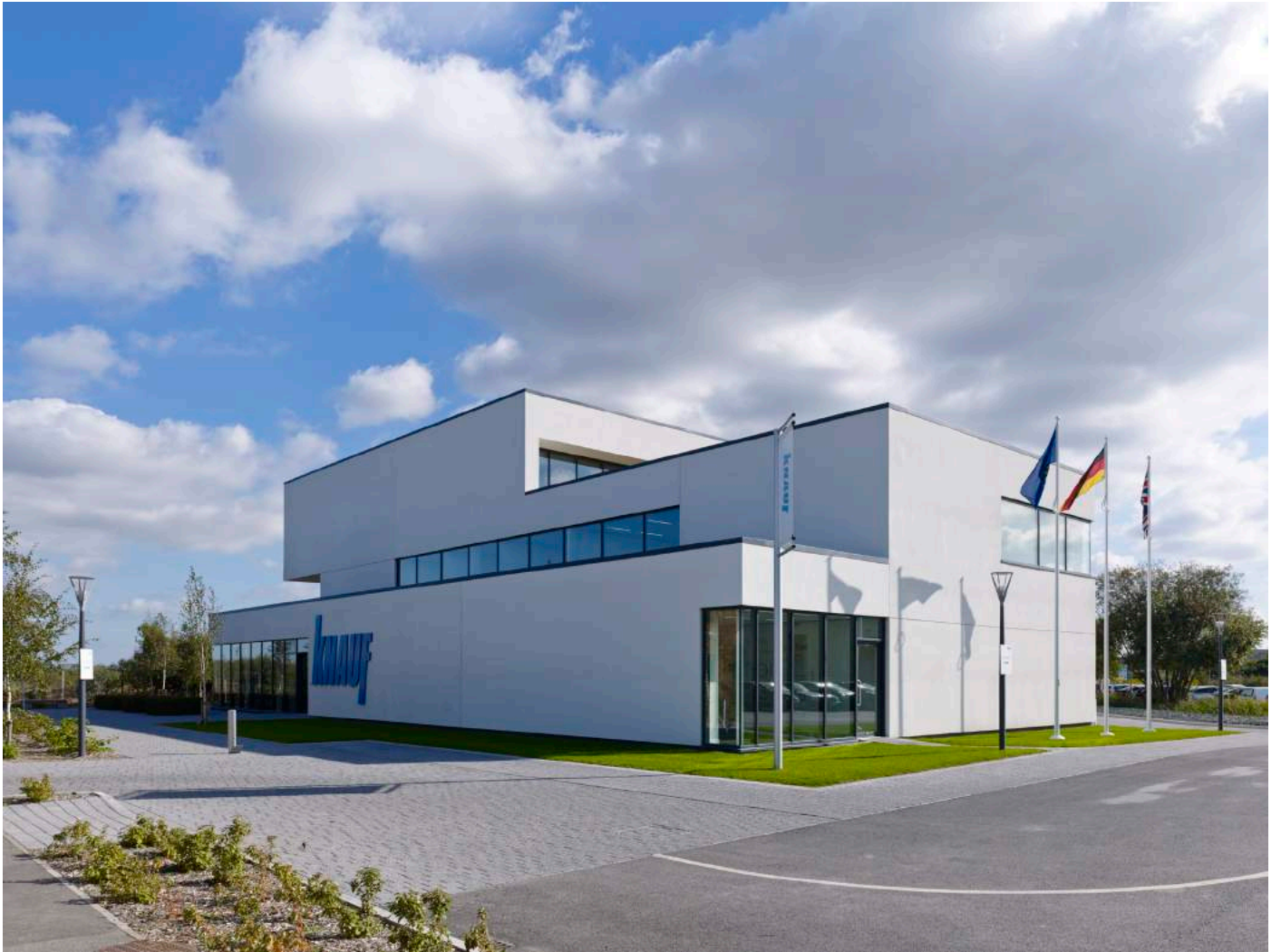
View into Piazza and Entrance
