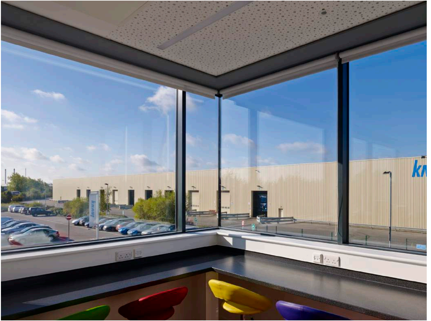
Staff area and manufacturing facility
