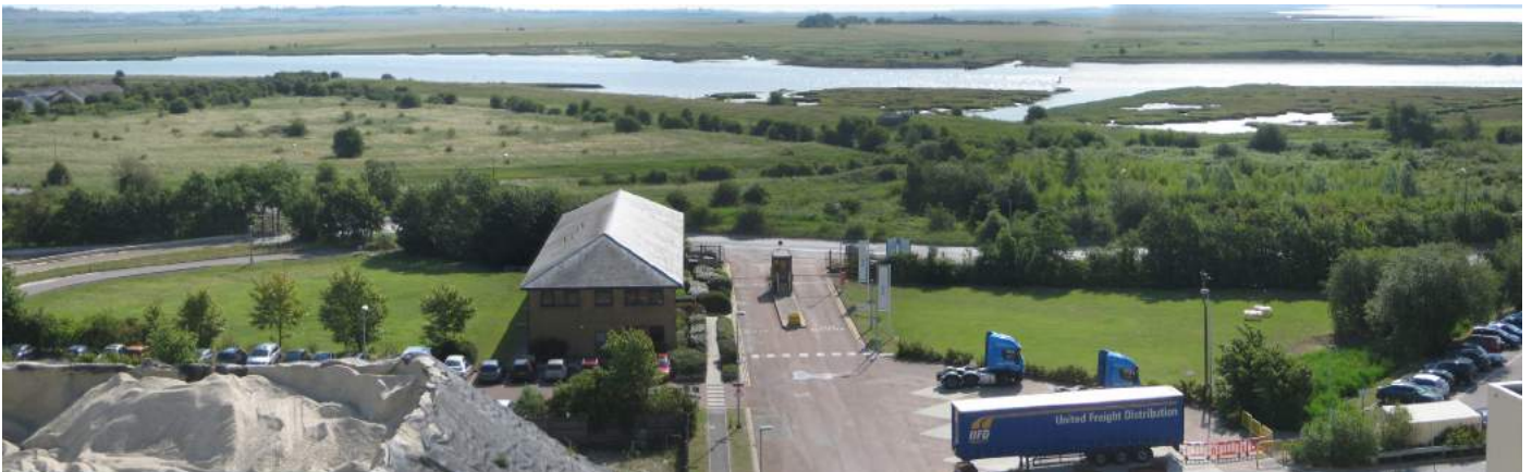
View over the swale and site
