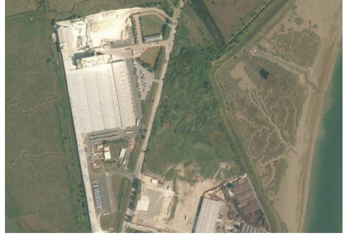
Aerial view of site. Extent of site outlined in red
