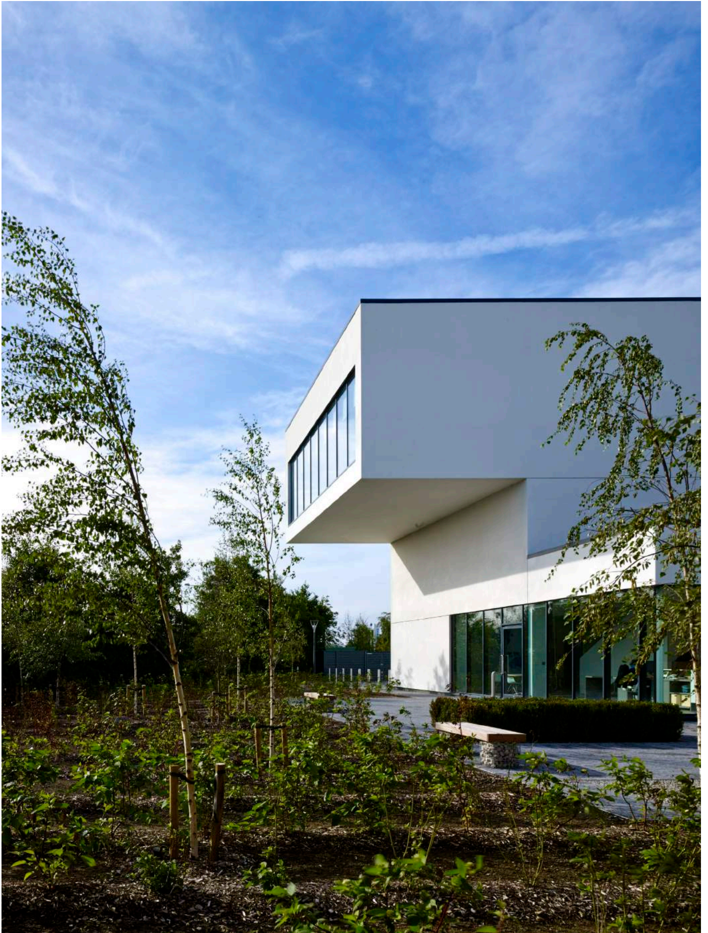
External courtyard and cantilever
